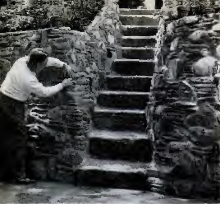
Wall of 2000 patterns was built around a terrace and steps. Each pattern consists of shale laid around a unique or colorful stone. Drainage holes keep wall dry
